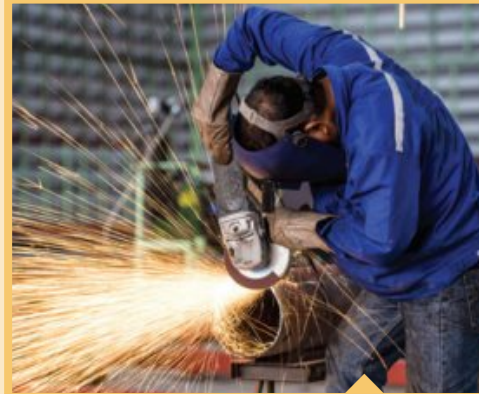
⊘ Workers exposed to lead
